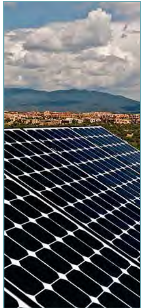
Photovoltaic collectors for producing electricity soak up the sun from the rooftop of this Santa Fe home. It has earned Platinum certification from LEED for Homes and Gold certification from Build Green New Mexico, the programs' highest ratings.
