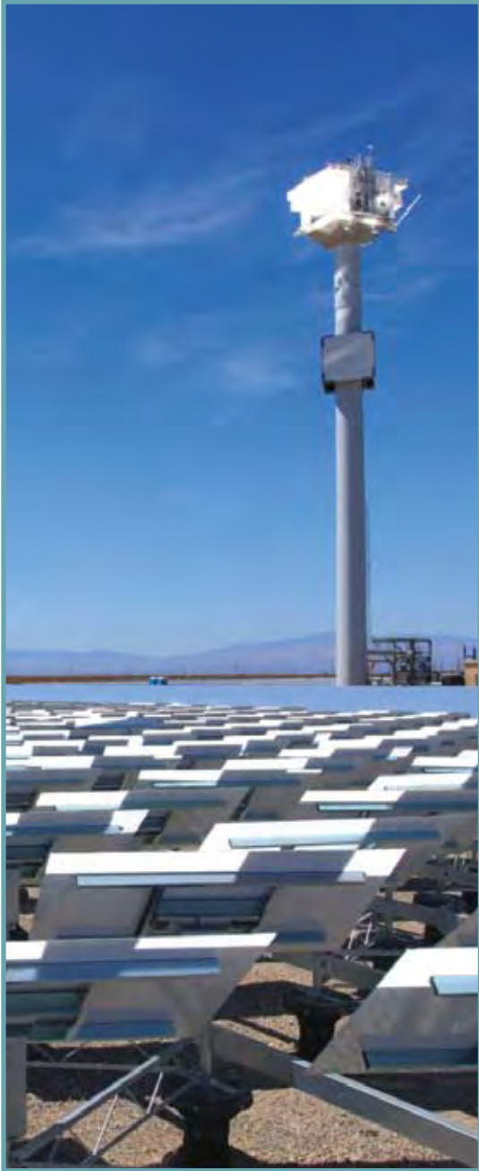
eSolar power plant technology utilizes small, flat mirrors which track the sun with high precision and reflect the sun's heat to a tower-mounted receiver, which boils water to create steam. This steam powers a traditional turbine and generator to produce solar electricity.
